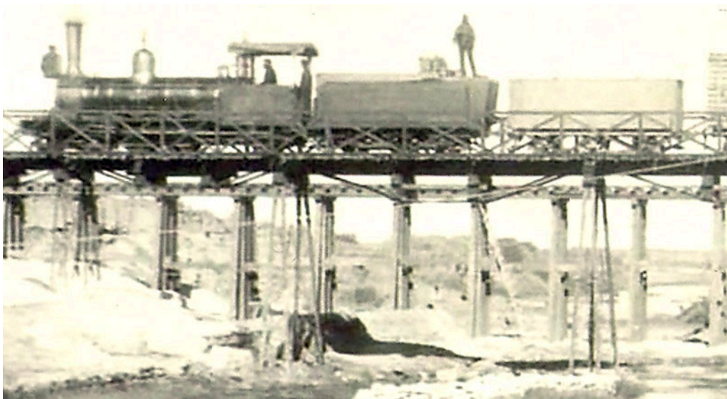
No. 27 'ASCOTAN' . Note the raised sides of the bunker, presumably to increase the capacity substantially.
