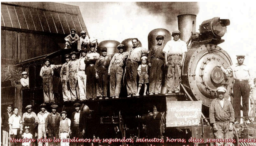
No. 41 at Maestranza Puquios in 1938, already with its rear sand-dome moved forward of the steam dome.
