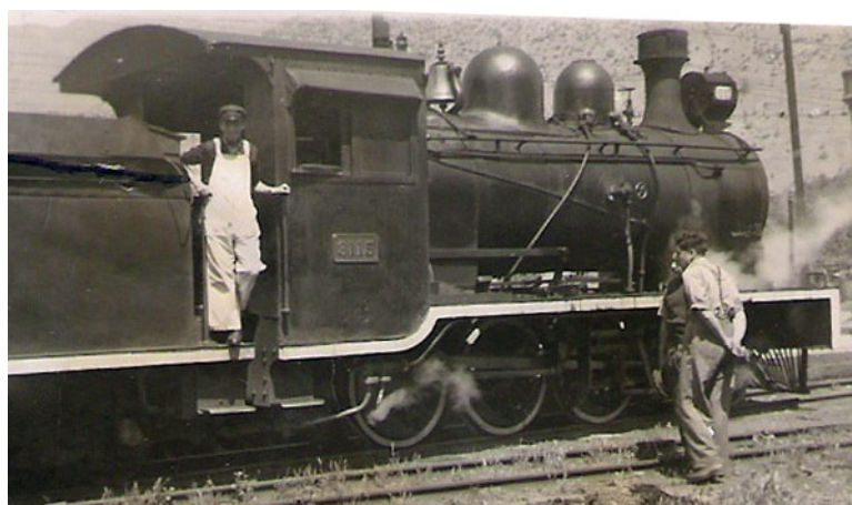
Tipo T no. 3115 . Note again that the air pump has been moved to the left side, possibly to improve sightlines for the drivers.
