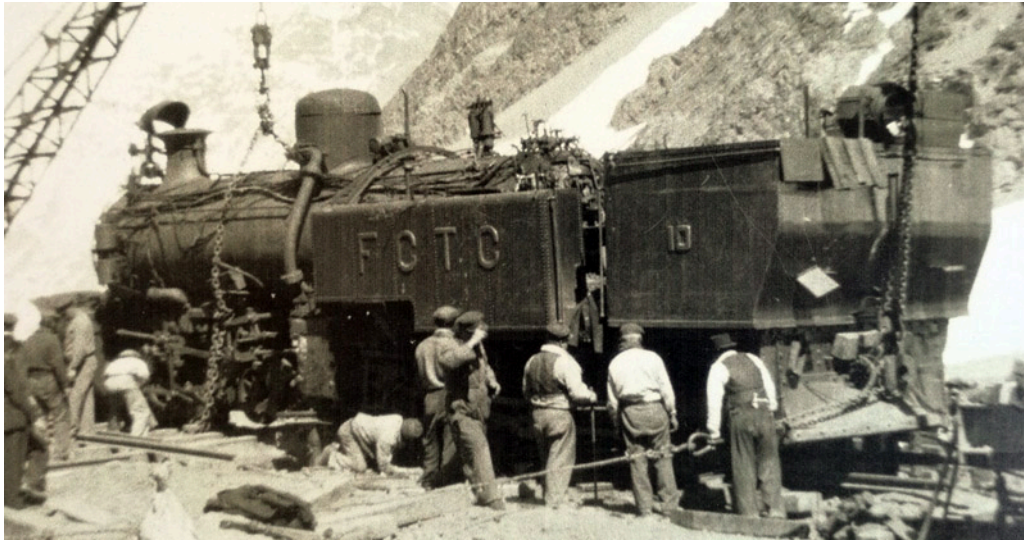
No. 10 , seen being recovered after a derailment in 1944, and with replacement tanks, having a long 'lower step' and a cab entrance immediately in front of the bunker. By that date the chimney has been shortened and has gained a moveable cowl.
