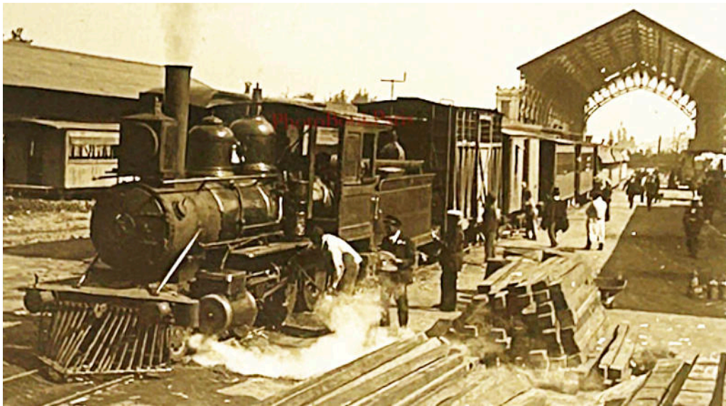
The positioning of the bell between the steam dome and the sand dome, and the domes both being lower than the cab roof, suggest that this was one of the four 2-6-0s. The location is uncertain. The Pirque terminus had an overall roof like this, but it had a closed end facing north. Photo provided by courtesy of Sr. Pablo Moraga.
