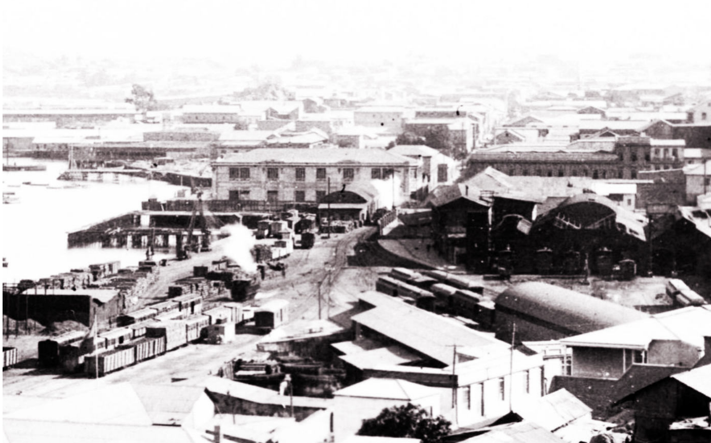
Coquimbo port station yard in mixed gauge days, with the loco shed over to the right. It would be good to find a better shot of this scene. The crowded nature of the site explains why the maestranza eventually moved to Ovalle.
