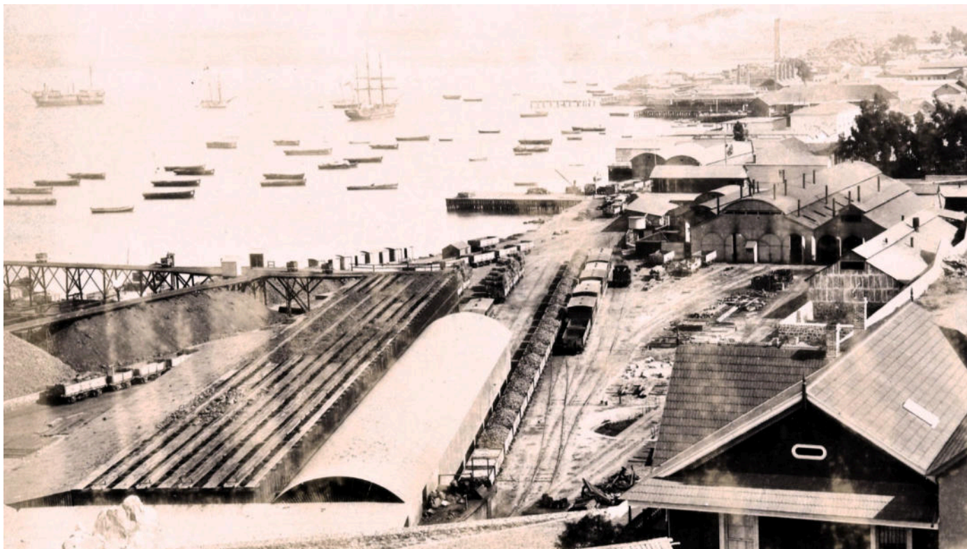
This earlier scene, in broad gauge days, was taken from a few yards further south than the other. The curved roof shed in the foreground was lower right in the
