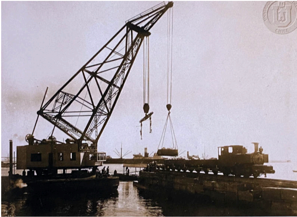
Bringing concrete blocks to be placed by a floating crane, 7 th May 1928.
