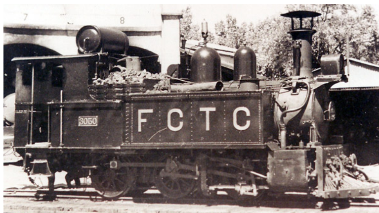
Photo courtesy of Jens Schindler. The engine is now air-braked, with a cylinder on the cab roof, and has a narrow sand-dome probably borrowed from some other type of loco.
