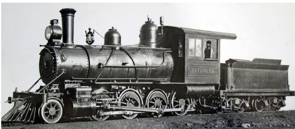
No. 19 'CATAPILCO' in almost original condition but with a slightly different cab, without the curved tops to the windows that were standard on this batch.
