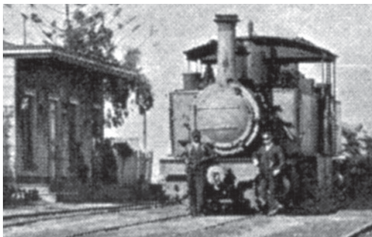
An unidentified Fairlie brings a freight into a wayside station, giving us an end-on view and showing the left-hung smokebox door common on the NRC. -----
