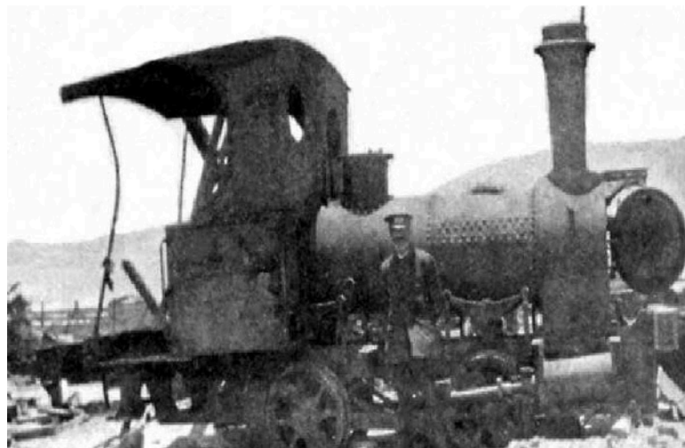
Photo from Señor Pablo Moraga's collection. Labelled as being at Chañaral and probably of this engine, despite there being differences from the drawing above. The chimney and dome are different, and the lower cabsides suggest that the tanks had been replaced. Boilers did not last long in the desert and a replacement might well have been slightly different.
