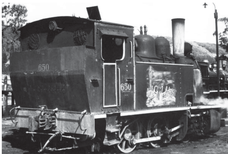
A photo by Ken Mills showing no. 650 , with a welded bunker and a slightly taller chimney than that shown above.
