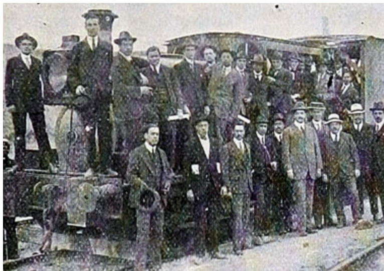
This 1915 photo, from Sucesos issue 680, seems to show one of these locos with minor modifications including the addition of dumb buffers and a large headlight. The visitors were engineering students from the University of Chile.
