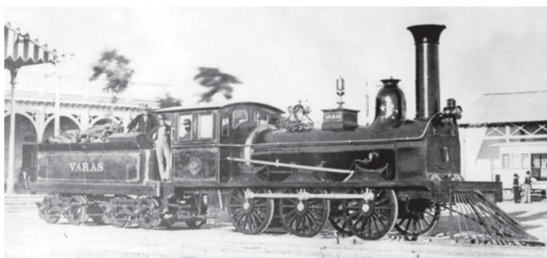
Note the much taller chimney, and the modified cab, when compared with the diagram above.
