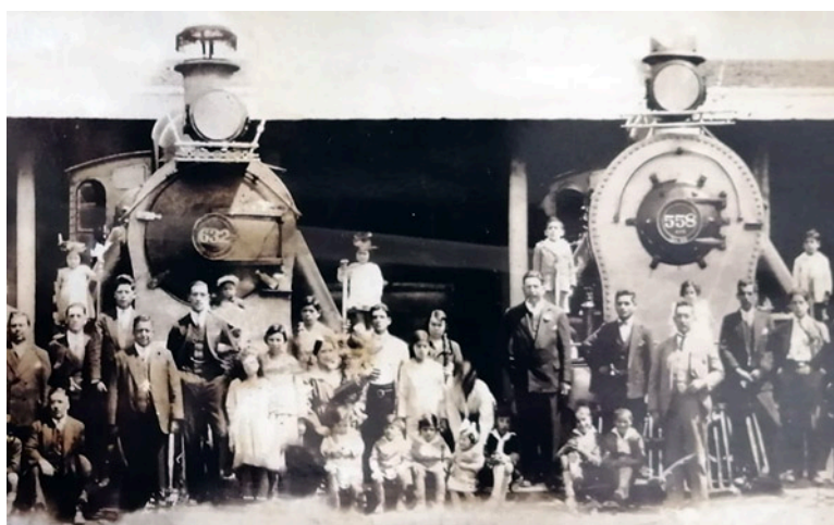
No. 632 , on the left is one of these locally-built tipo 57 engines still with a large smokebox door, presumably as built, whilst tipo 58 no. 558 on the right has a US-style small smokebox door.
