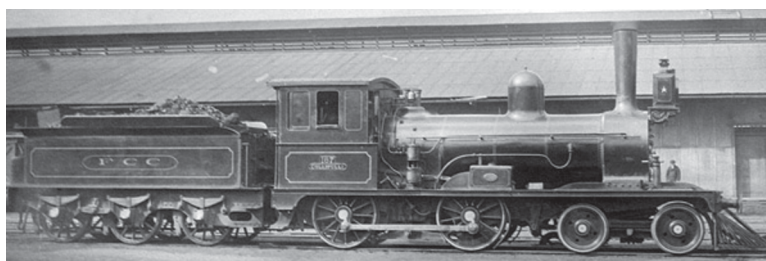
No. 167 'COLLIPULLI' after rebuilding with a longer fixed wheelbase and also a longer cab.
